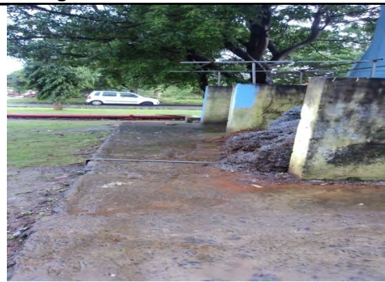
Shutter right side After cleaning
